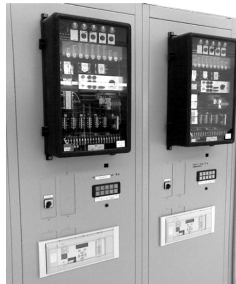
Fig. 1. Fragment of the protection panel at a distance of crucial lines 161 kV containing electromechanical relays of LZ31 type (above) included for working in parallel with an MPD type MiCOM P437 (below)
